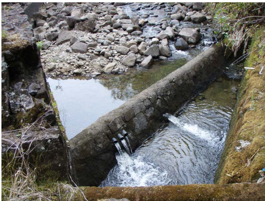
Figure 5-27. Diversion downstream of site 5 and taken on the right side facing upstream. (6/30/2009; Tributary name: Honomanū (64009004); PBN: ln005p-009-063009; Surveyor: Nishiura, L.; SBN: ln005d-063009; Lat. (DD): 20.83271, Long. (DD): -156.18056).
